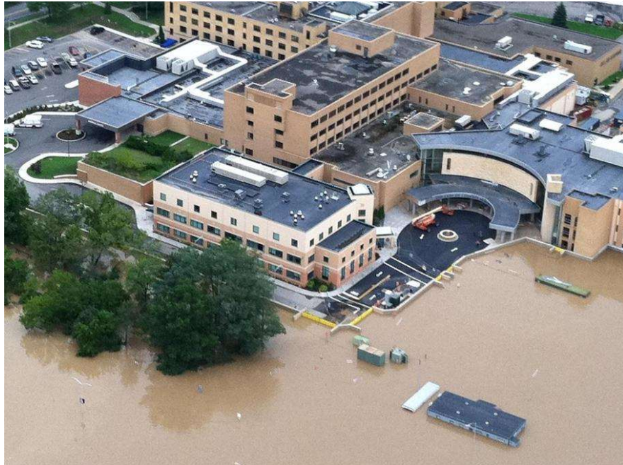
Figure 6.1. Floodwall protecting Our Lady of Lourdes Hospital in Binghamton, New York. FEMA.
