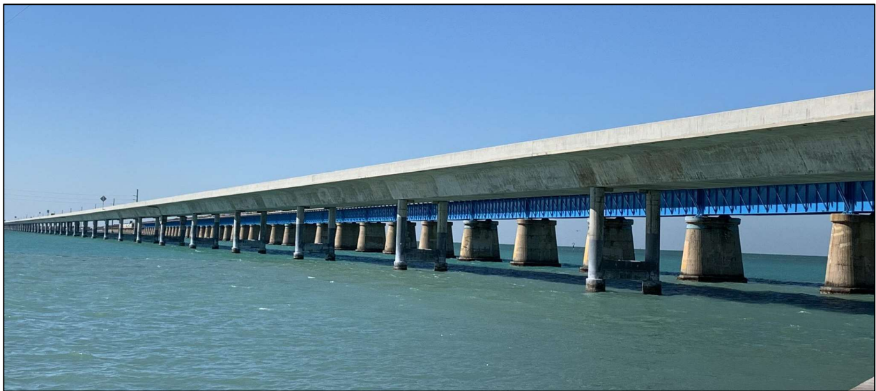
Figure 1.2. Seven Mile Bridge south of Marathon representing the southern boundary of the Middle Keys. Photo: Shoreline Conservation Initiative.
