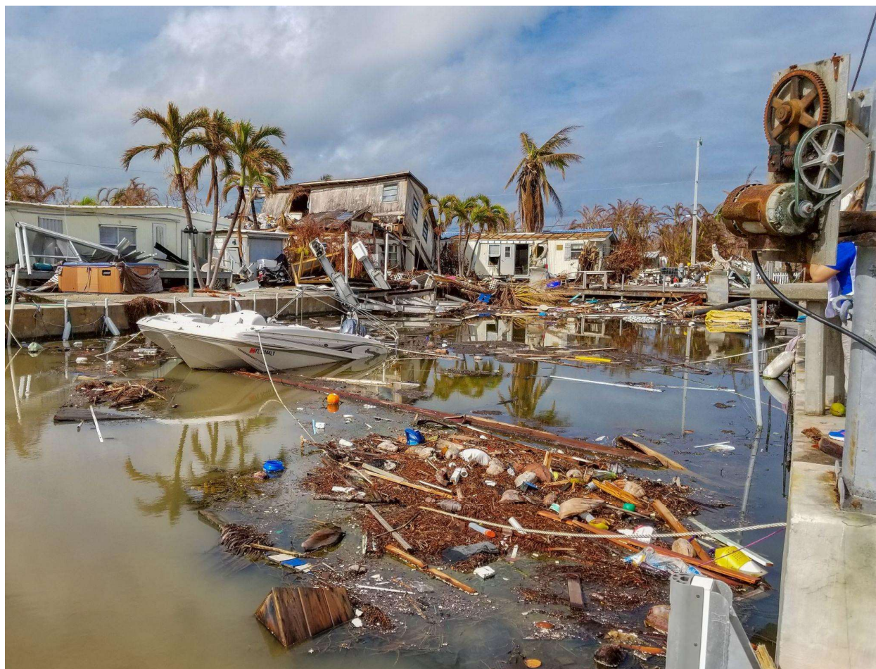
Figure 2.3. Debris littering a canal in the Florida Keys after hurricane Irma. Photo: https://www.monroecounty-fl.gov/ .
