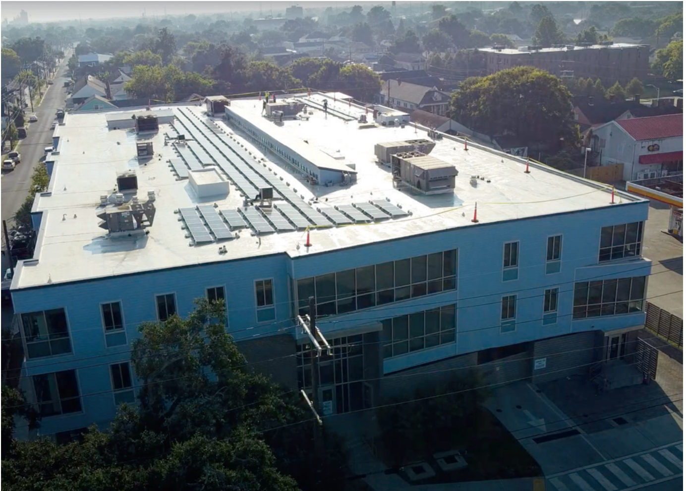
CrescentCare facility in Louisiana with solar panels installed.
